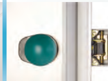
emergency internal door release is easily operated even when the door is locked
